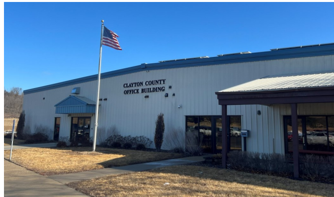
Clayton County Office Building with new solar panels
